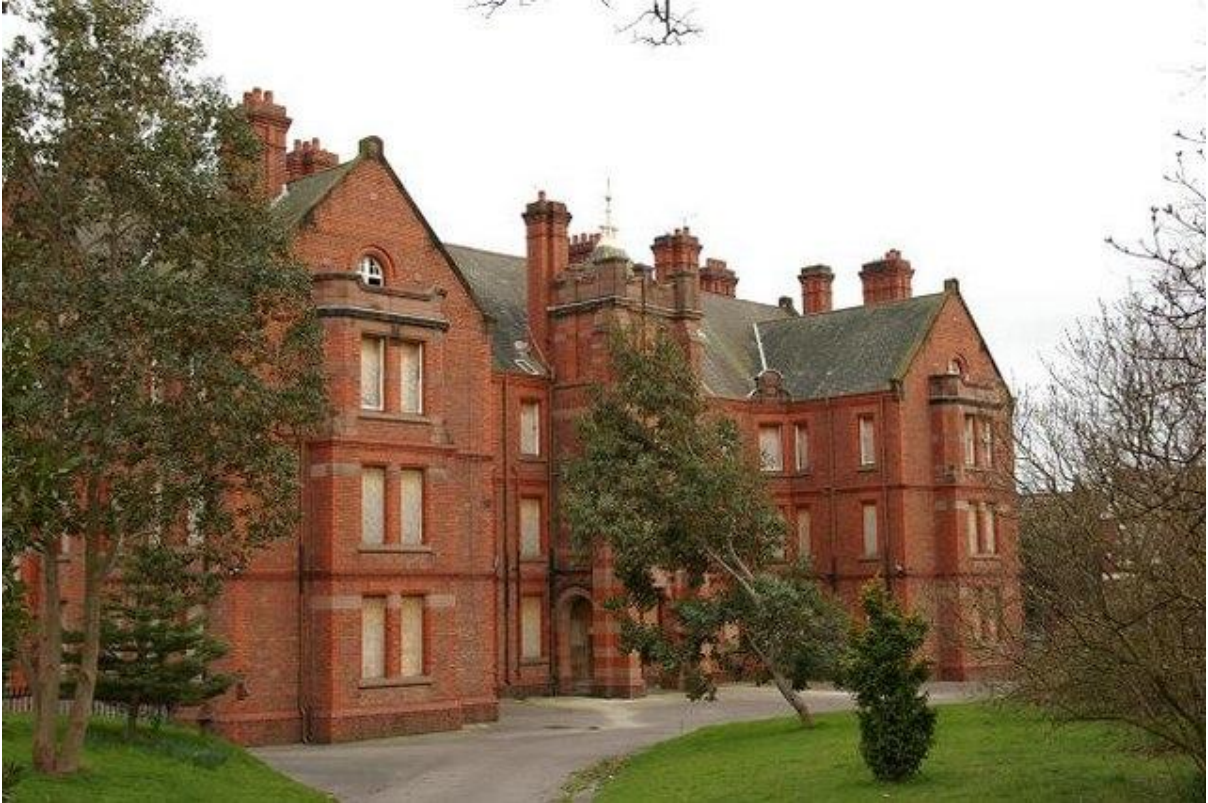
The main entrance and driveway of Andrew Gibson House, © Copyright Peter Craine and licensed under this Creative Commons Licence .
